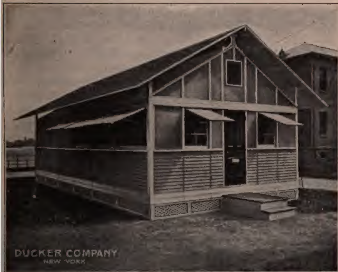
FIG. 203.— Portable hospital pavilion with double roof and double floor, system Ducker.
